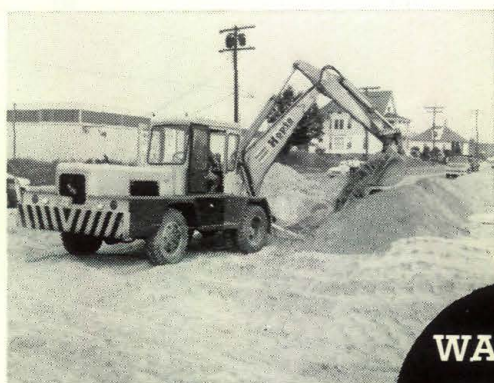
The Hopto® 200 hydraulic backhoe digging for gas lines.
