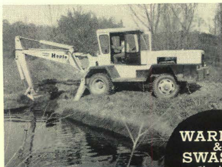
The Hopto® hydraulic backhoe digging a drainage trench for a southern construction company.
